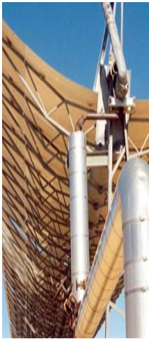
Concentrated Solar Power
